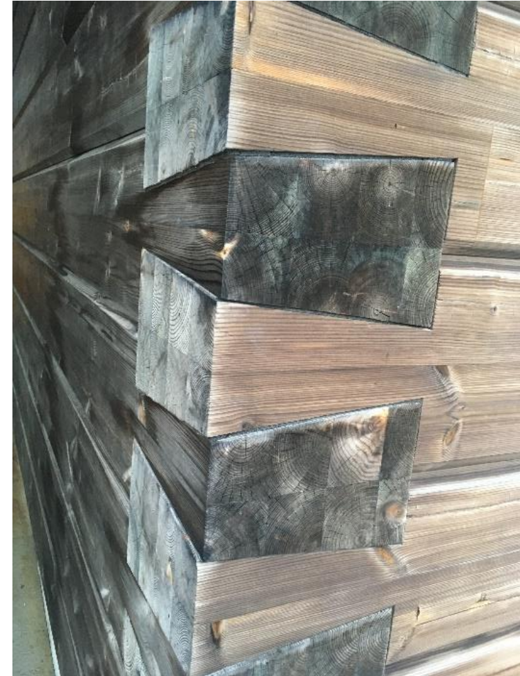
Traditional dovetail joint
