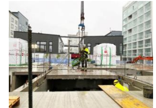
Assembly of reclaimed elements
