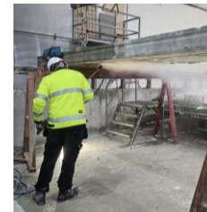
Refurbishment of elements
