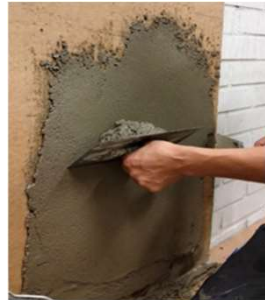
Savirappaus/ palonsuojalaasti (ECOSAFE, STALK)
